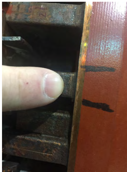
Figure 8: One of Several Fractured Rotor Bars Found During Shop Inspection
